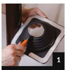
Select an appropriate Master Flash® Multi-Flash with a pipe range that goes below and beyond fitting. If necessary, follow the lines clearly shown on the flashing and create an opening 20-30% smaller than pipe diameter.
