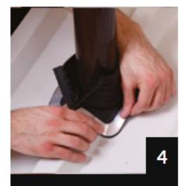
Press Master Flash® Multi-Flash down, bending it to conform to roof profile or irregularities. A blunt tool will help to form flashing to tight roof angles.
