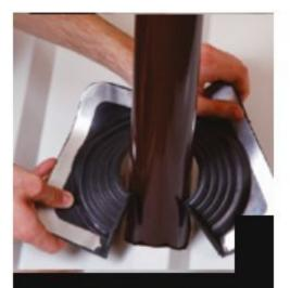
Slide the Master Flash® Multi-Flash down the pipe, using a nonpetroleum-based lubricant to ease installation. For Retrofit applications, wrap the product around the pipe.
