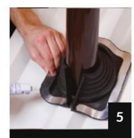
Apply sealant between the base of the flashing and the roof, as well as at the top of the flange.
